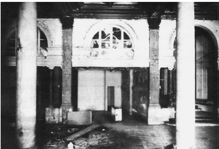
Figure 11. These dramatic "before" and "after" photographs show a severely deteriorated space restored to its original elegance: plaster has been repaired and painted; the scagliola columns have been restored to match marble using traditional craft techniques and missing decorative metalwork has been reinstalled in front of the windows. Although some reorganization of the space took place, notably the relocation of the front desk, the overall historic character of the space has been preserved. These views are of the lobby in the Willard Hotel, Washington, D.C. Credit: Commercial Photographers (left); Carol M. Highsmith (right)
