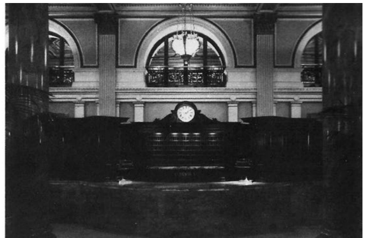
Figure 11. These dramatic "before" and "after" photographs show a severely deteriorated space restored to its original elegance: plaster has been repaired and painted; the scagliola columns have been restored to match marble using traditional craft techniques and missing decorative metalwork has been reinstalled in front of the windows. Although some reorganization of the space took place, notably the relocation of the front desk, the overall historic character of the space has been preserved. These views are of the lobby in the Willard Hotel, Washington, D.C. Credit: Commercial Photographers (left); Carol M. Highsmith (right)
