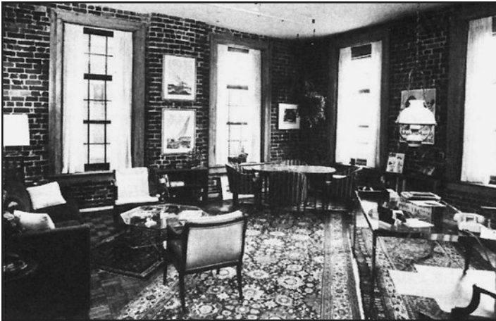
Figure 10. In this case plaster has been removed from perimeter walls, leaving brick exposed. In removing finishes from historic masonry walls, not only is there a loss of historic finish, but raw, unfinished walls are exposed, giving the interior an appearance it never had. Here, the exposed brick is of poor quality and the mortar joints are wide and badly struck. Plaster should have been retained and repaired, as necessary.
