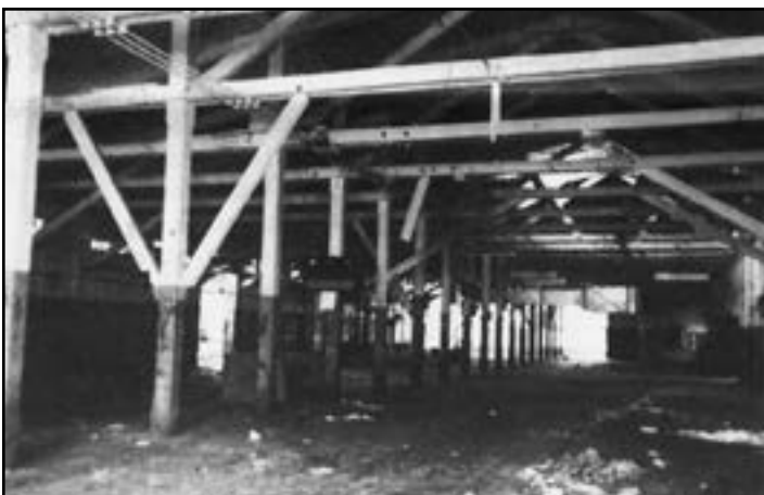
Figure 2. The interiors of mills and industrial buildings frequently are open, unadorned spaces with exposed structural elements. While the new uses to which this space could be put are many retail, residential, or office—the generous floor-to-ceiling height and exposed truss system are important character-defining features and should be retained in the process of rehabilitation.
